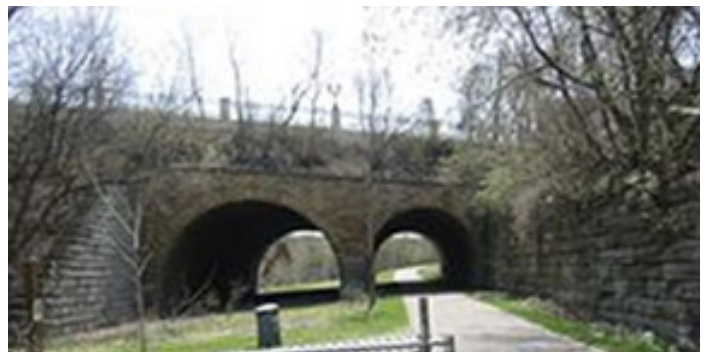
Seventh Street Bridge Improvement Arches 1884, St Paul, MN
