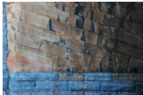
Helicoid coursing in the oblique barrel vault at St. Paul MN
