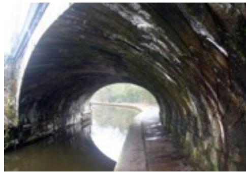
Peter Robinson, Logarithmic Skew Arch, Bridge 74A, Leeds and Liverpool Canal
