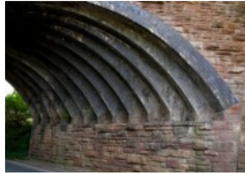
Ledbury & Gloucester Railway, Ribbed Arch, Hereford Road Bridge, Ledbury
