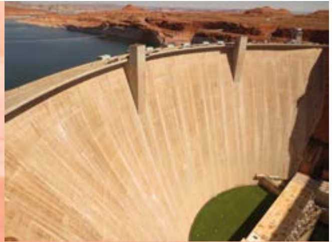
Continuous 24 hr cement placement over 3 years
