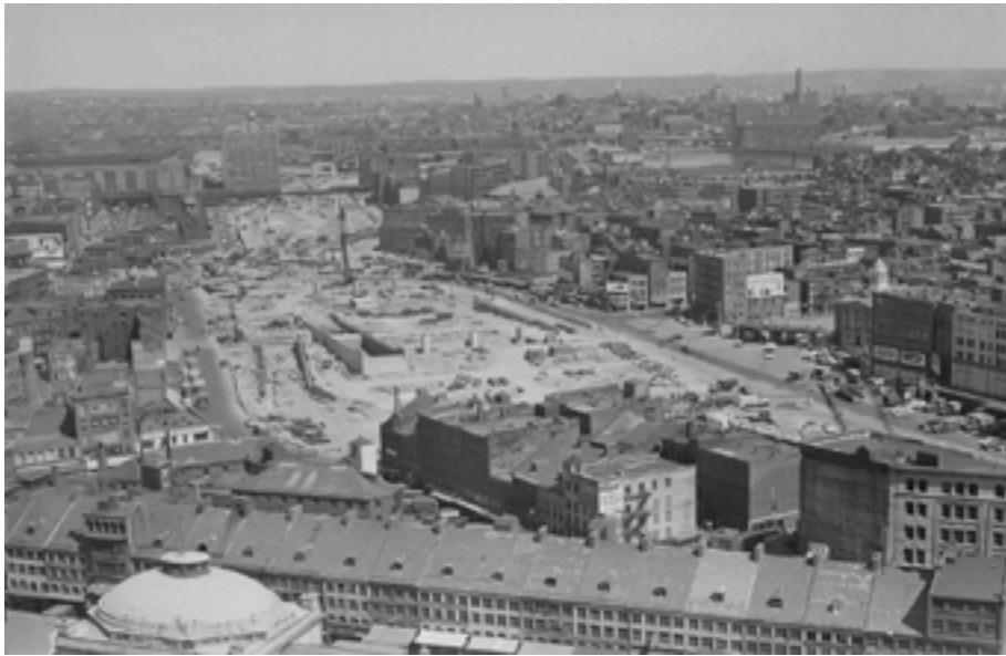
Central Artery project clearance - Boston (Wermiel)
