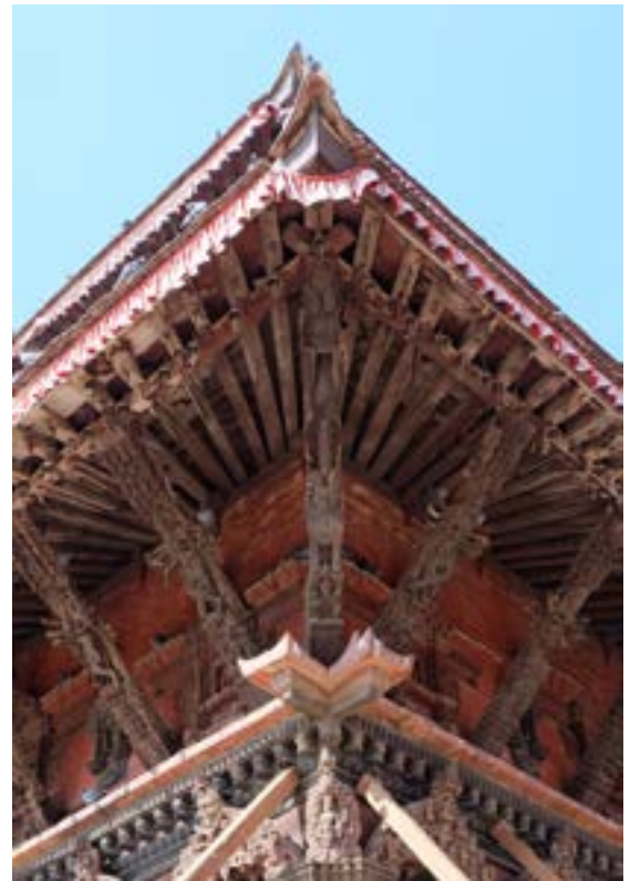
Absence of a rigid Timber – Strut joint at the Vishwanath Temple, Patan Durbar Square
