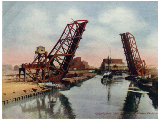
Jack Knife Bridge over Chicago River
