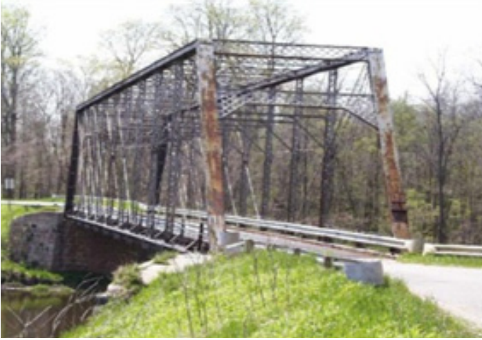
Figure 2. Charlotte Highway bridge at its original location (Source: http://www.historicbridges.org/bridges/browser/?bridgebrowser=truss/charlotte/ )
