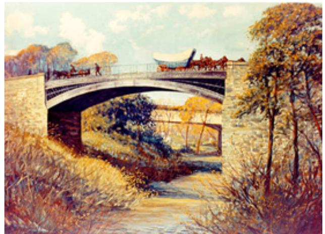
*First iron bridge in the United States, Dunlap's Creek, PA, 80ft span*
