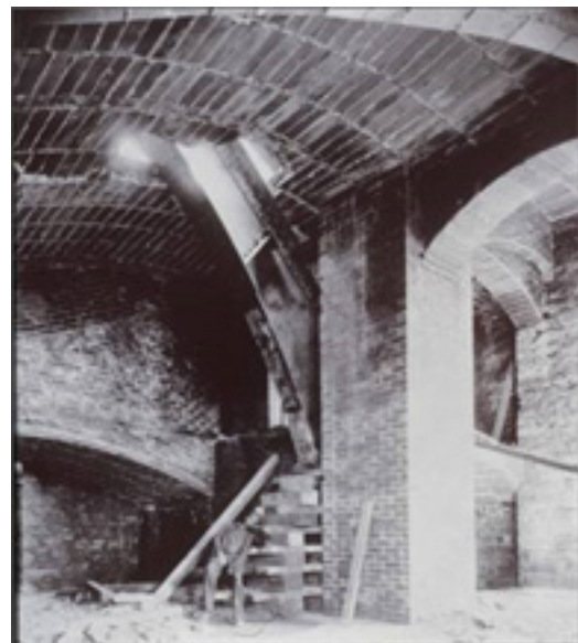
Collapsed beam – University of Virginia
