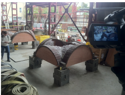
Completed vault at end of workshop
