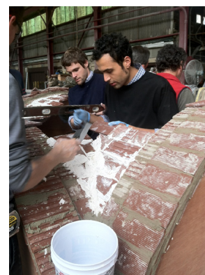
Gabriel Pardo Redondo, APTI and CHSA member, working on a Guastavino vault
