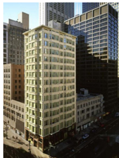
Burnham Hotel, Chicago. (Old Reliance Building)
