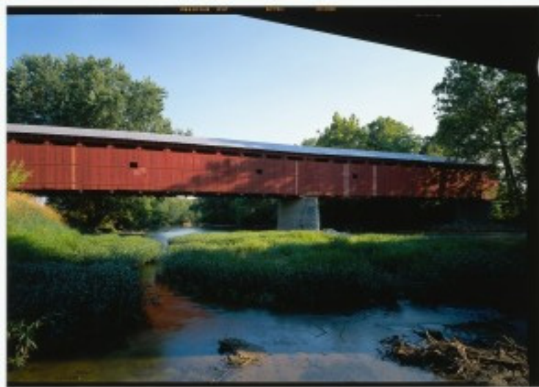
Eldean Bridge (Long Truss, 1860) in Miami County, will be on both Saturday tours. HAER photo by Jet Lowe
