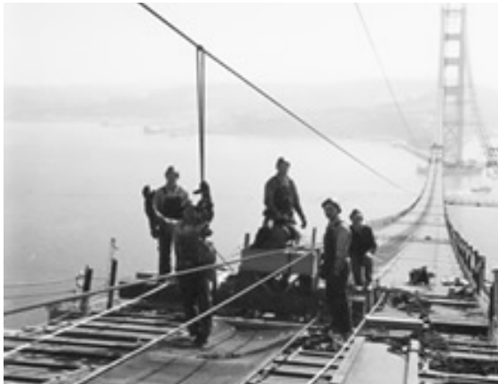
Main Cable Spinning
