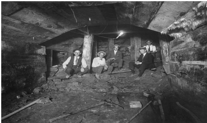
Mr. Whiting Directing Tunnel Project in Baltimore
